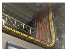
**Our locking tray:** No more zip ties mean faster installation, less plastic waste, and no risk of ties dropping into your production area causing a mess or even worse, a shutdown.
