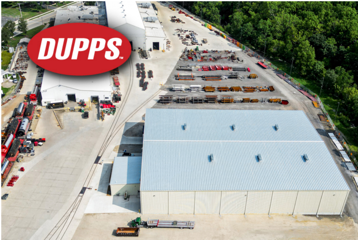
The Dupps Company's new 48,000 sq. ft. state-of-the-art manufacturing center.
